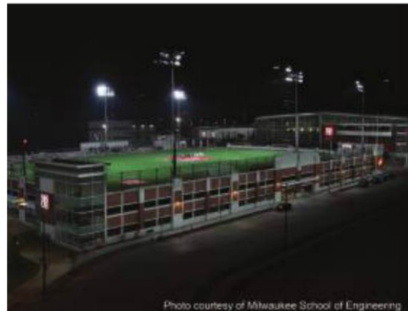
Photo courtesy of Milwaukee School of Engineering
