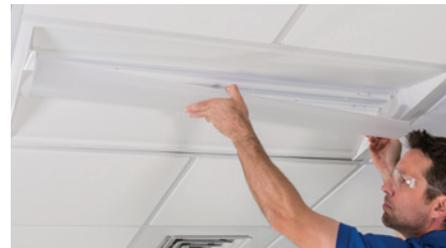
Install the lens over the LEDs, inserting the lens' flat edges over the sides of the bracket, pushing the middle of the lens.
