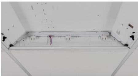
Cut the power wires going into the input side of the ballast. The ballast may remain in place, unless it needs to be removed for extra clearance or local code compliance.
