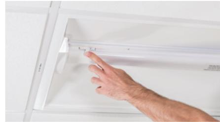
Secure the latches, ensuring they've made a proper connection.
