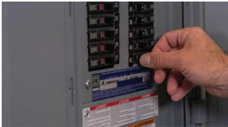
Disconnect the power to the light fixture you're replacing.
