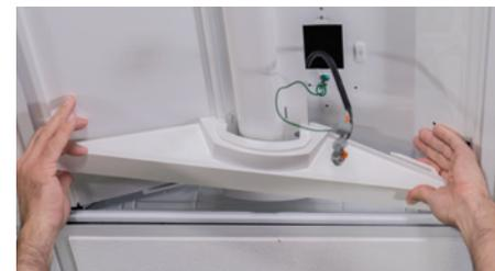
While holding on to the retrofit main assembly, insert the corner of the end cap into the corner of the existing troffer pan and the T-Grid Ceiling assembly.
