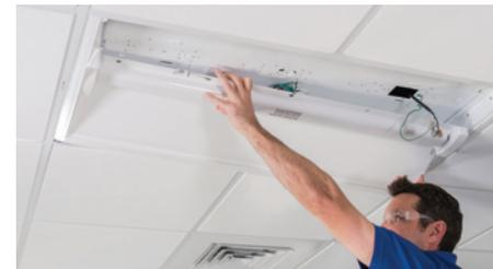
Then slide the other end of the main assembly into the existing troffer pan. Gently push the full main assembly up into the pan, making sure the end cap is flush with the ceiling grid and there are no gaps.
