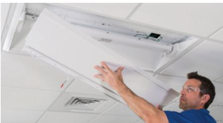
Bring the retrofit side panel up to the existing troffer pan and connect the ground wire on the back of the side panel retrofit main assembly. Then snap it into the supplied space.
