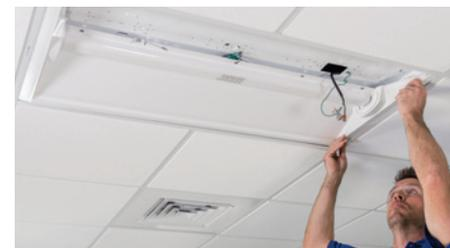
Attach the sliding end cap over the retrofit main assembly bracket. Then slide the other end of the sliding end cap into place, ensuring there are no gaps.
