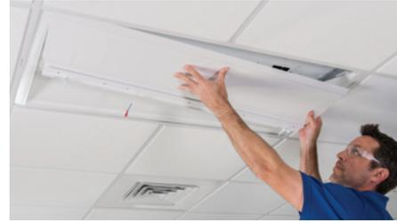
Insert the edge of the side panel opposite the latches between the existing troffer panel and the T-Grid Assembly. Then insert the other side to the top of the main assembly by engaging the 2 latches on the side panel into the slots provided.
