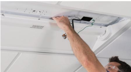
To avoid pinching, make sure the wires are tucked on top of the main assembly and that no wires are exposed.
