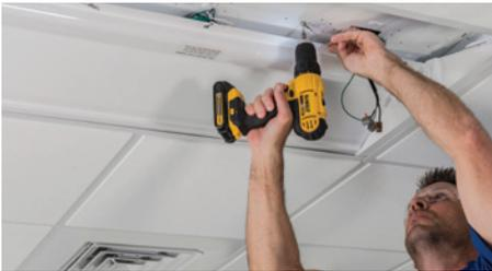
Attach one end of each safety cable to the top of the existing troffer pan using the supplied self-drilling screws.
