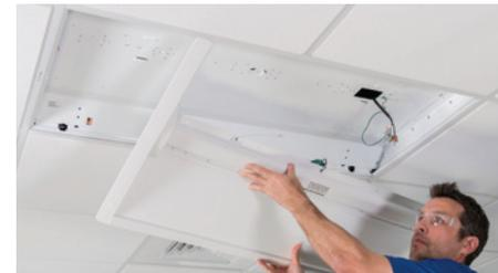
Bring the retrofit main assembly into the existing troffer pan at an angle. Insert the corner of the main assembly into the corner between the existing pan and the T-Grid ceiling.
