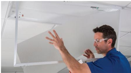
Remove the existing fluorescent parts from the pan, including the prismatic or parabolic lens, door, fluorescent tubes and cover. Removal of the lamp holders is optional.
